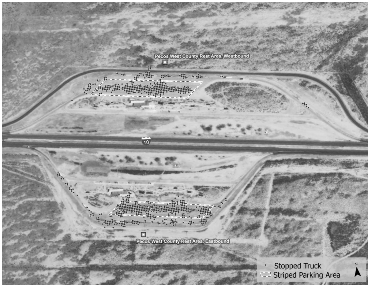
Figure 12: Parking Inside and Outside of Striped Locations
